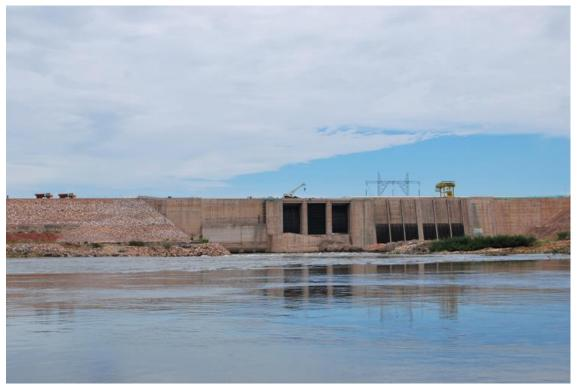
The Sinop Dam seen from the upstream side with the river at its natural level without a dam. The three spillway gates, and the two sets of three stop-logs at the intakes of the two turbines, are all located at depths that would draw water below the level of the
