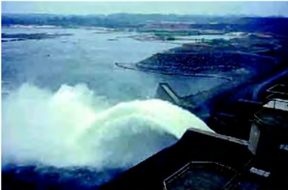
Figure 1. Spillway of the Tucuruí Dam, in the Tocantins River, state of Pará. Water leaves the reservoir at a depth of 20m, where it carried great quantities of methane. Pulverization in the form of droplets releases this greenhouse gas in the atmosphere, contributing to global warming. (Photograph by Philip M. Fearnside).
