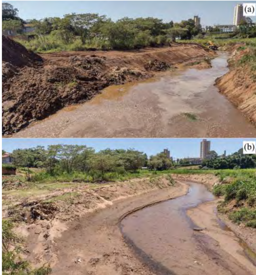
139 Figure 1. A silted stream: (a) during; and (b) after intervention in its APPs. 140 141
